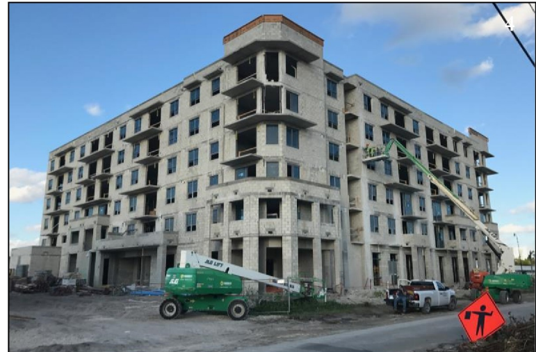
(4) Site Photo of Building #4 at Hallandale ArtSquare
